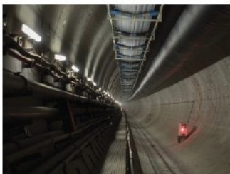
Northolt tunnel: new milestone
